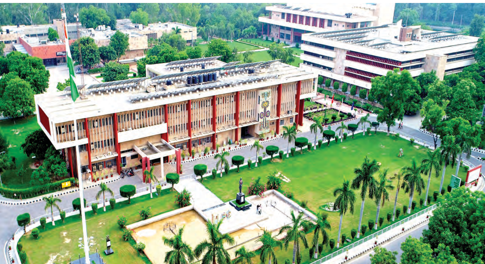
Aerial view of Fletcher Bhawan of CCSHAU Hisar
